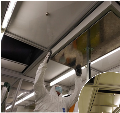
Technician installing a FFU in a DTU cleanroom.
