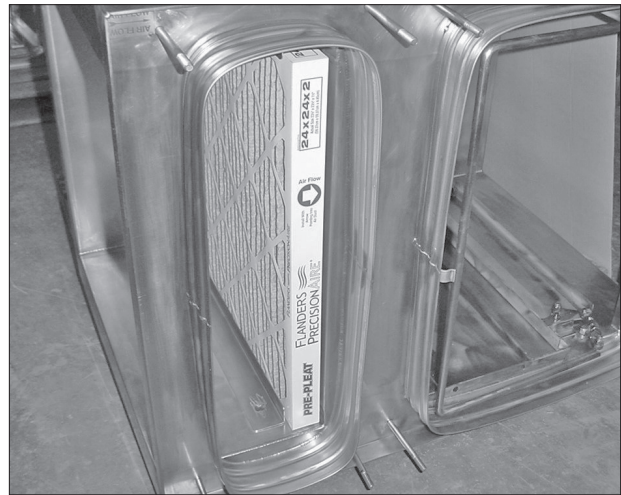
Filter Removal Rods Are Standard on BF-Series, Ordered as Optional on KF-Series
